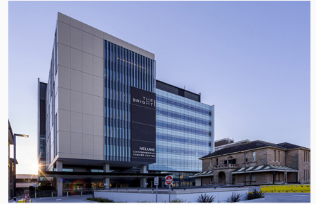
The Bright Alliance Building - Prince Of Wales Cancer Centre
